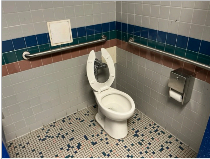
TOILET STALL OVERVIEW
