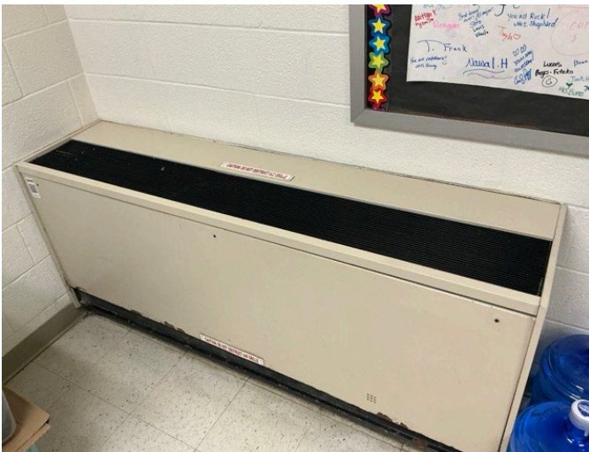
21 - TYPICAL UNIT VENTILATOR
